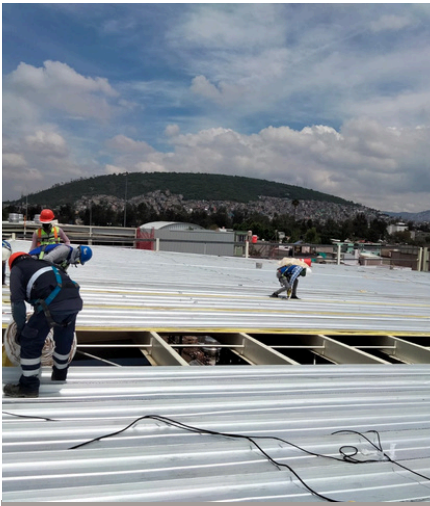
BODEGA INDUSTRIAL - PEASA
